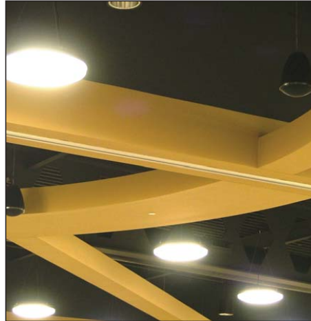
The speakers in the main convention center were selected because they were designed specifically for open-truss ceilings. There are 32 speakers in this area.
